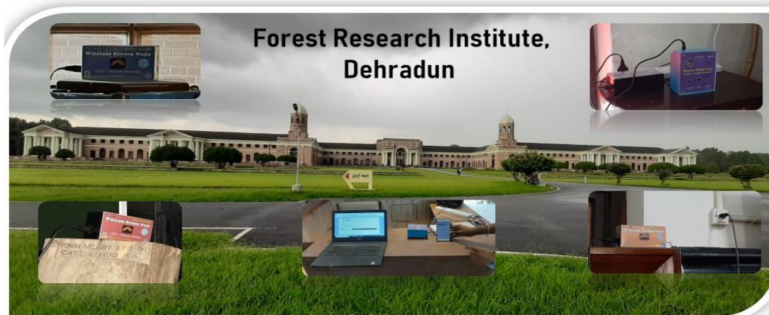
Installation of developed system at various rooms of FRI for initial studies
