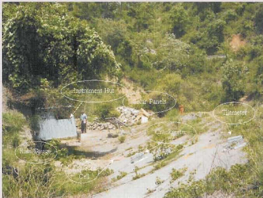
A View of Landslide Monitoring System installed at Mansa Devi (Haridwar)
