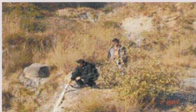
Installation of the System
